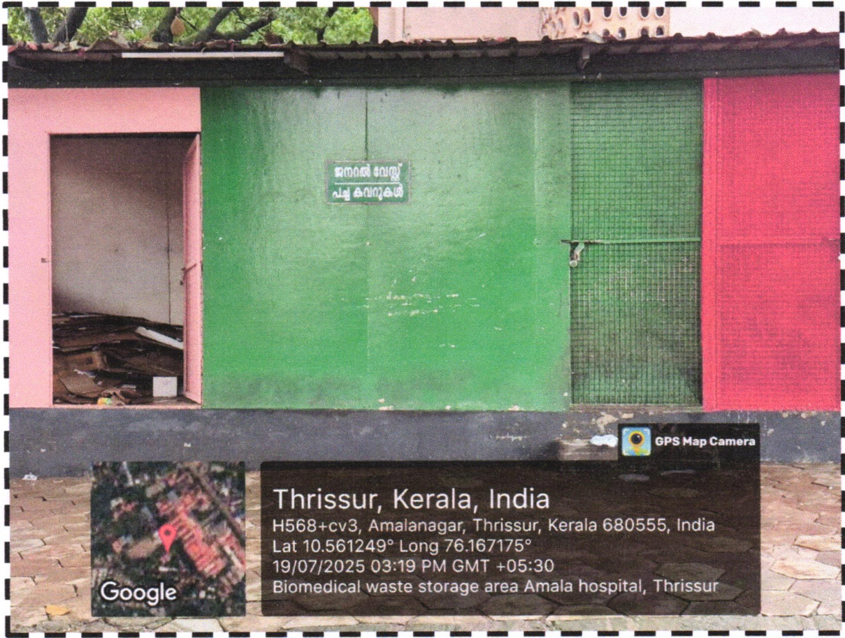
GENERAL WASTE STORAGE AREA
