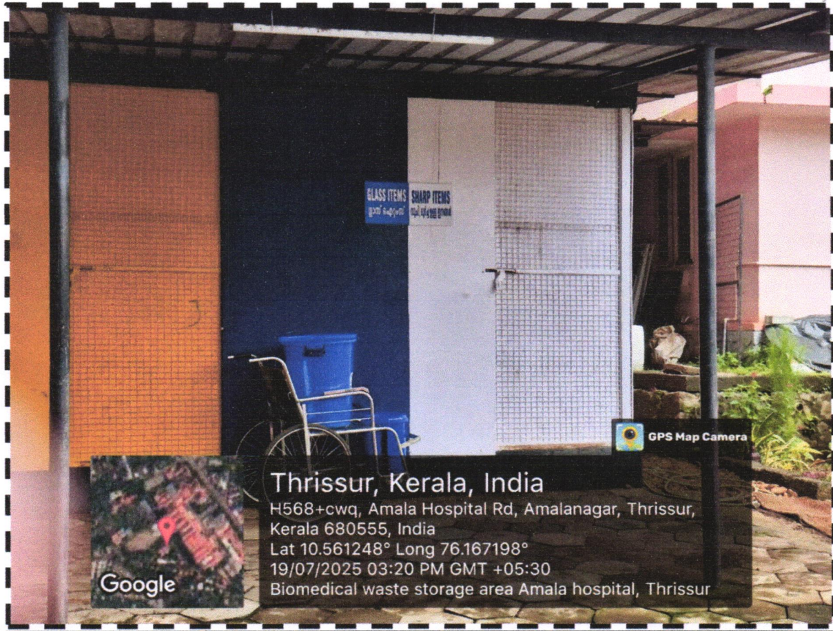
STORAGE AREA FOR GLASS ITEMS AND SHARP ITEMS
